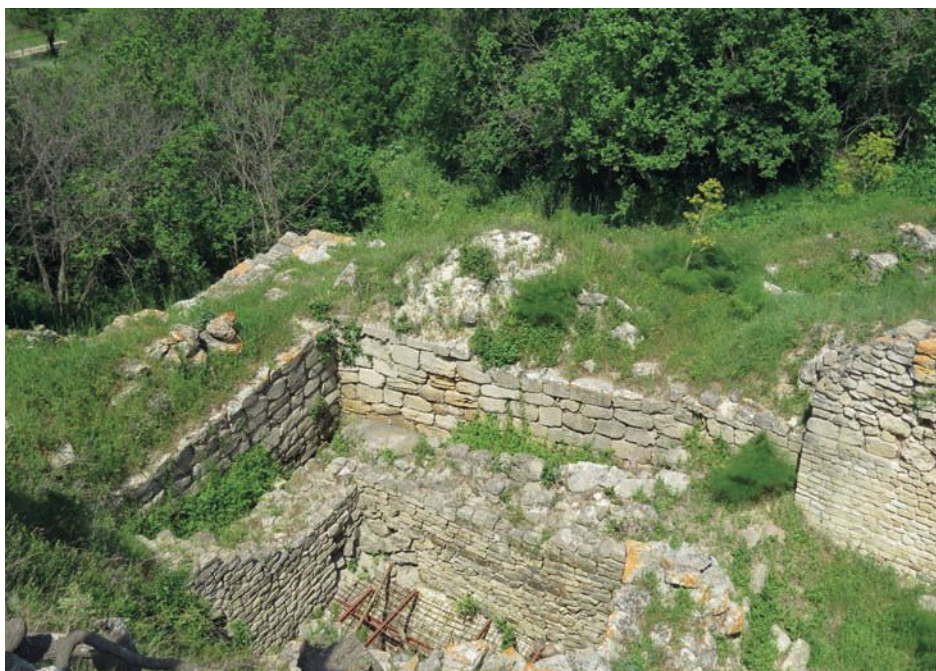
The walls help visitors to visualise the thriving cities of Troy (there were at least seven) that were built, destroyed and rebuilt on this ancient site in Western Turkey. Photograph © Diana Bentley.
