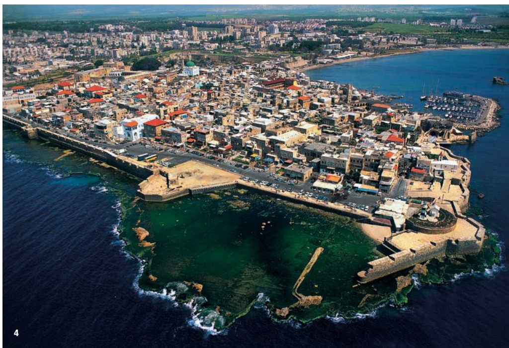
4. Aerial view of the Old City and fortress of Akko, jutting into the Mediterranean.
